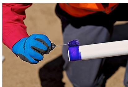
In cold weather, solvent cements penetrate and soften the surfaces of plastic pipe and fittings more slowly than in warm weather. The plastic is also more resistant to solvent attack. Therefore, it is very important to pre-soften surfaces with an aggressive primer. A longer cure time is necessary due to a slower evaporation rate in cold weather.
